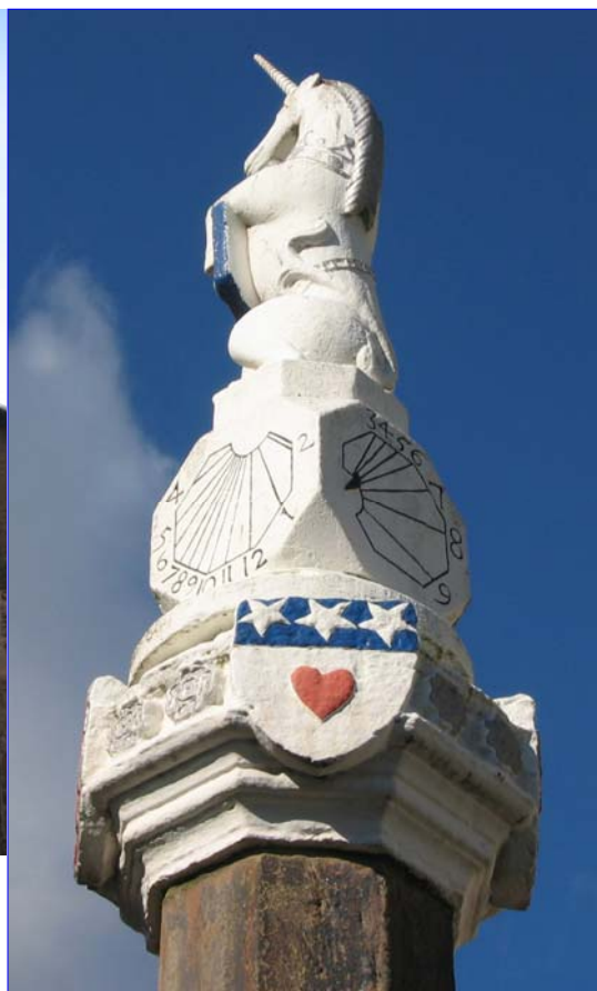
Figs 6, 7 & 8. The Inverkeithing Cross. Although Ross’s drawing seems to indicate a direct south face, the photograph shows the dials do not face the cardinal directions but decline significantly,
