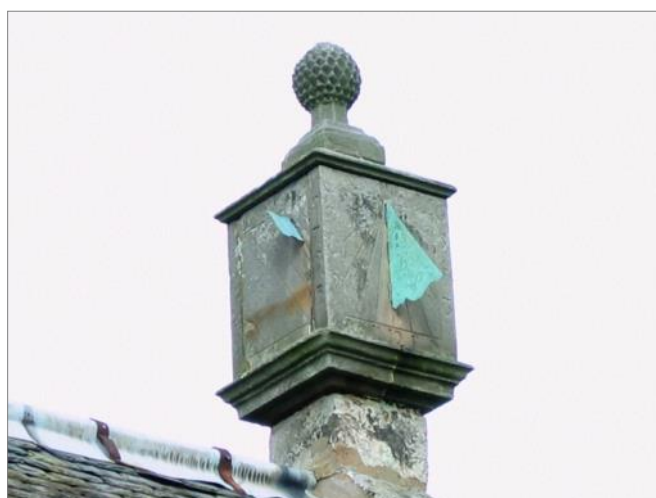
Figs 7 and 8. The cube dial at Pencaitland church. Above: the south and east faces; below: the south and west faces.
