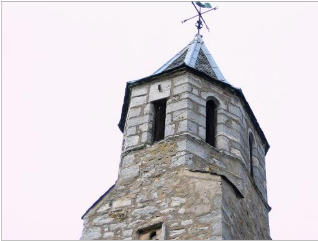
Fig. 9. The dial on the tower at Pencaitland church.
